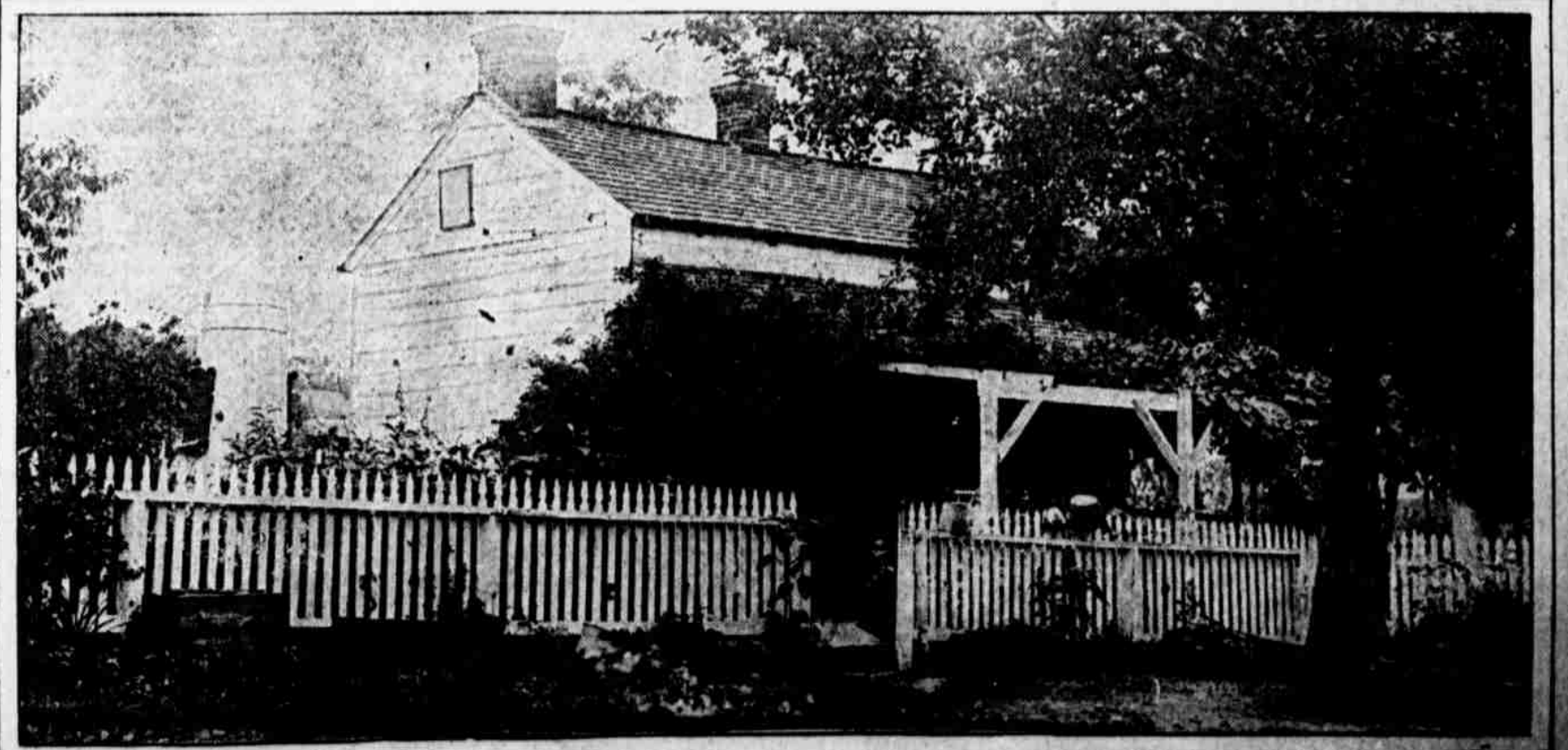
HOUSE WHERE GENERAL MEADE HAD HEADQUARTERS DURING THE BATTLE This building, still standing, is one of the hallowed landmarks of a town that bristles with reminders of the Civil War's greatest engagement. The commander who successfully led the Union troops against Lee's invaders of Pennsylvania soil, it will be remembered, was a Pennsylvanian.
