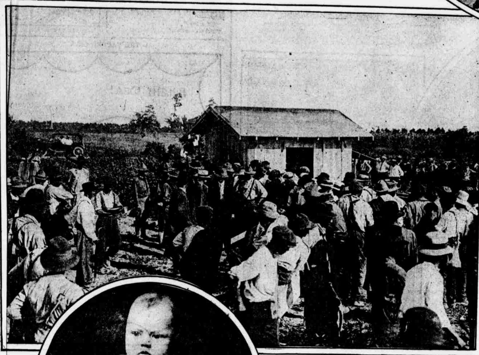
PAYDAY AT CAMP HANCOCK, NEAR AUGUSTA, GA. THE SHORTAGE OF LABOR HAS SERIOUSLY HANDICAPPED THE WORK OF PREPARING THIS CANTONMENT FOR THE COMING OF PENNSYLVANIA'S NATIONAL GUARDSMEN
