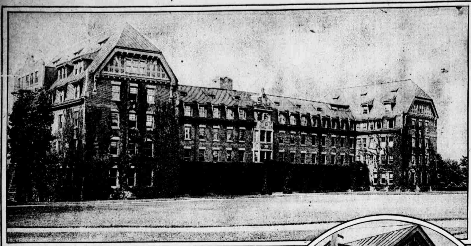
POTTSTOWN IS KNOWN EDUCATIONALLY AS THE HOME OF THE HILL SCHOOL The ivy-mantled structure is the main hall of the school. In the curriculum of the Hill School is included a splendid course in the rudiments of military training.
