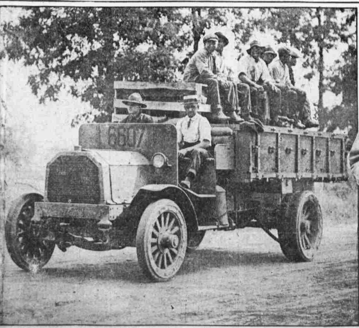
A CONSTANT STREAM OF TRUCKS LOADED WITH BUILDING MATERIAL Hums along the Jersey roads in the direction of the camp site bearing the components out of which the great army garrison is to be constructed.
