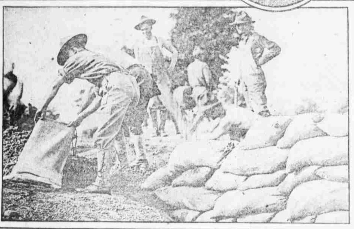
ERECTING A BARRIAGE OF SANDBAGS AT THE FORT MYER TRAINING CAMP. Recruits for the Officers' Reserve Corps from New Jersey and Delaware are rapidly acquiring one of the rudiments of field warfare, that a soldier's first duty is to take care of his own safety when in the presence of the enemy.
