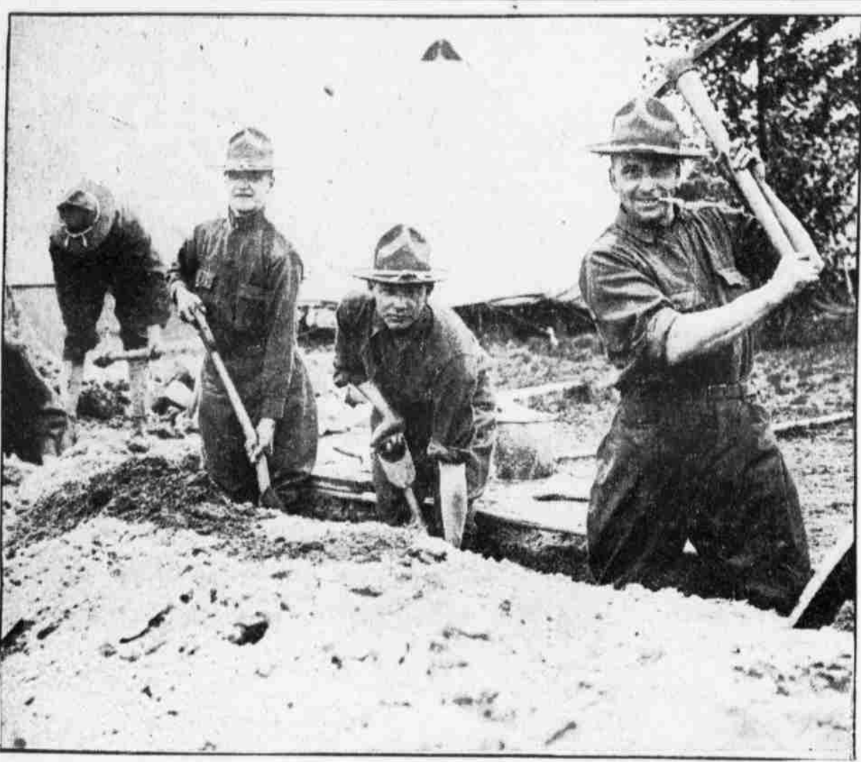
AT WORK IN THE TRENCHES IN CAMDEN
