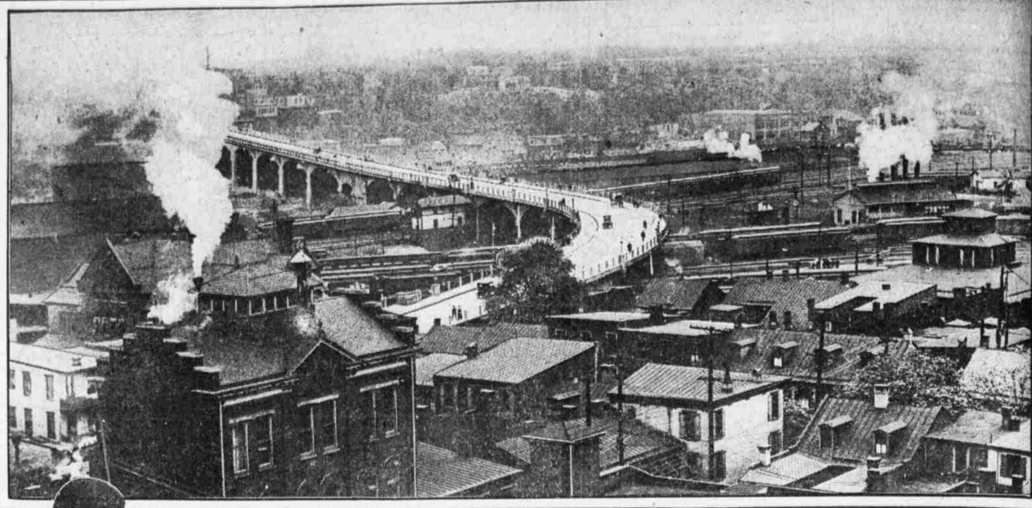
GENERAL VIEW OF THE MULBERRY STREET BRIDGE WHERE IT CROSSES THE NETWORK OF TRACKS OF THE PENNSYLVANIA AND READING RAILROAD SYSTEMS, WITH NORTH HARRISBURG RISING UP IN THE DISTANCE
