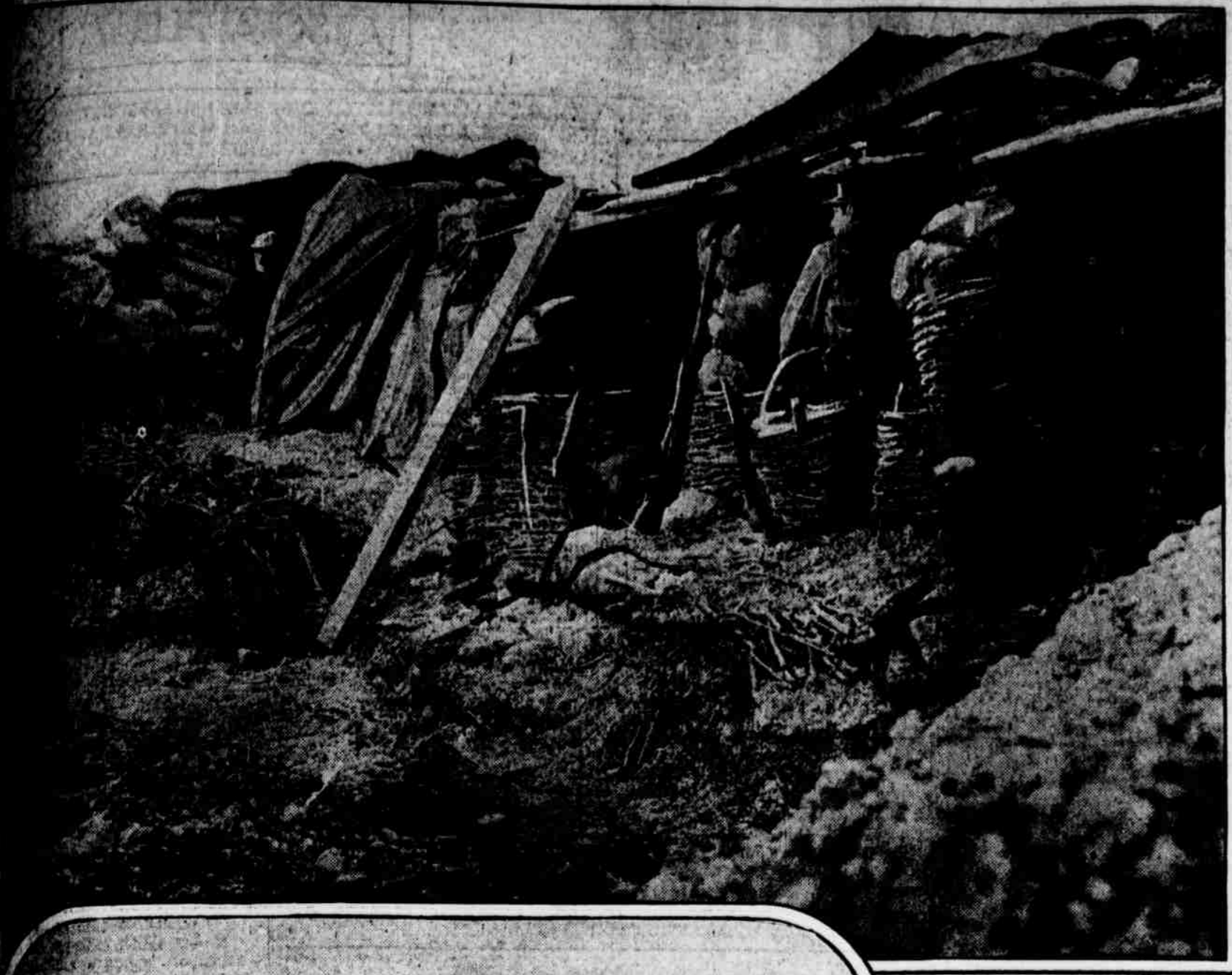
Copyright Public Ledger Company. GERMAN FORTIFICATIONS BEFORE NESLE, TAKEN ONE HOUR AFTER FRENCH OCCUPATION
