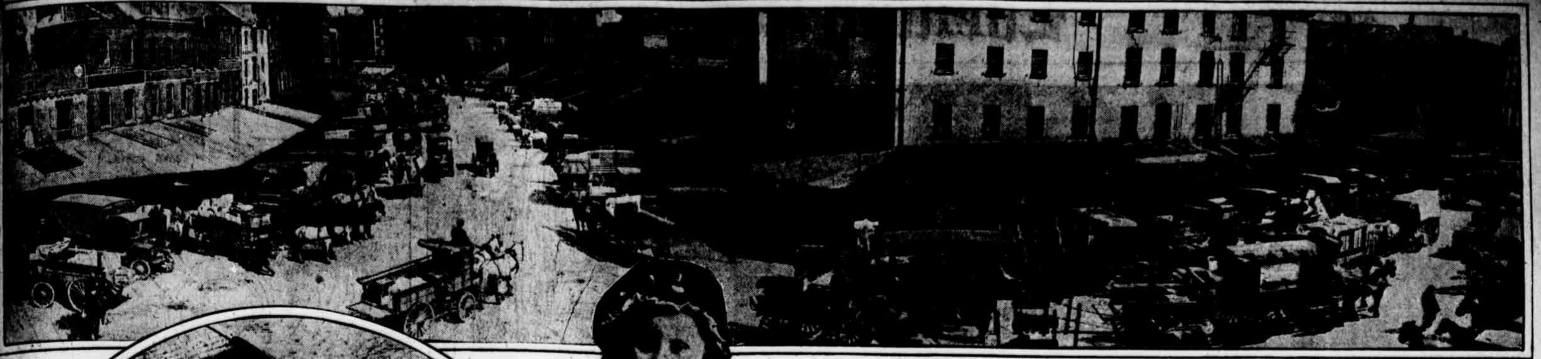
THESE ARE BUSY DAYS IN DOCK STREET AS THE EARLY SPRING VEGETABLES APPEAR. The produce district still clings to the horse for delivery purposes, even on the heaviest market days.
