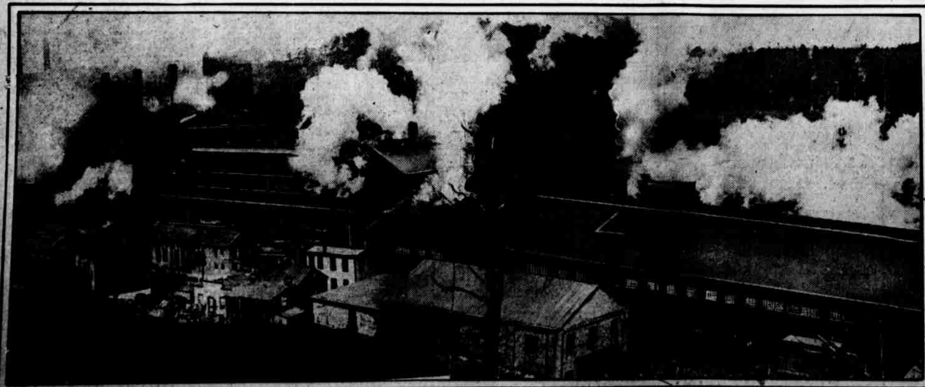
SUGGESTING A TRANSPLANTED BIT OF SMOKY PITTSBURGH The Eastern Steel Works, employing a small army of workmen, contributes millions yearly in taxes to Pottsville residents.
