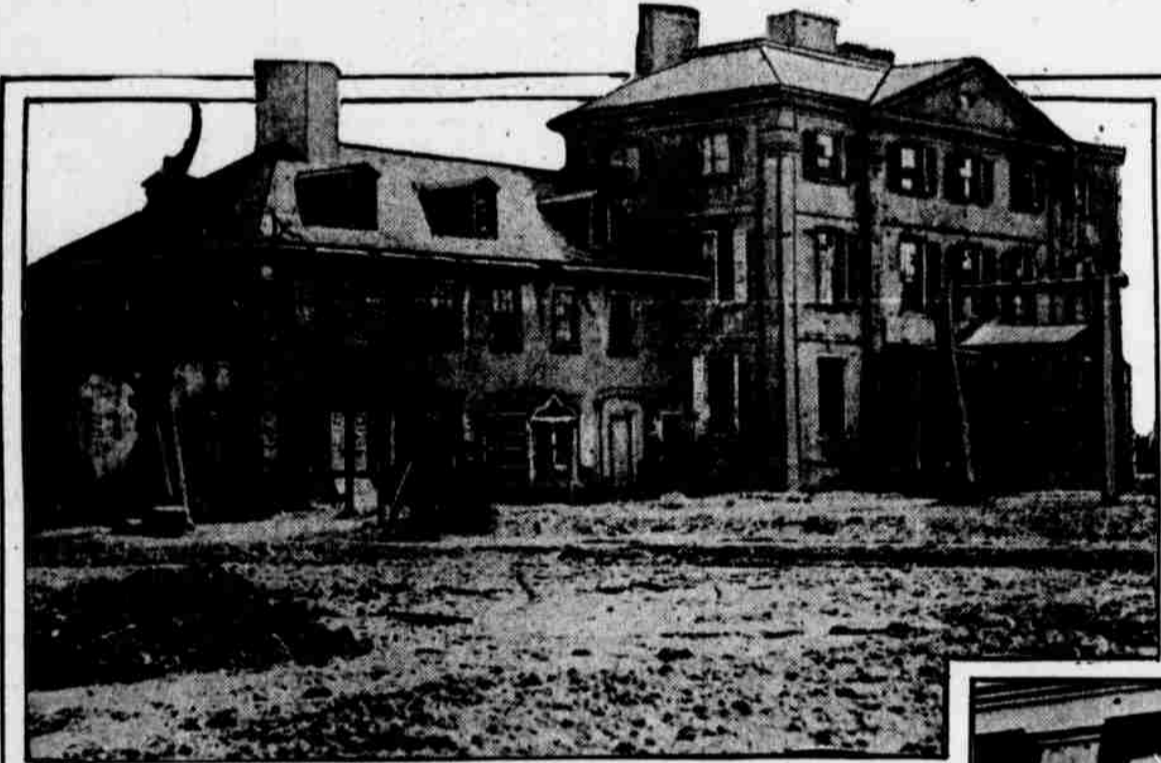
PROGRESS DOOMS FRANKFORD LANDMARK Chalkley Hall, on Wheatsteeff lane, is to be torn down to give way to a manufacturing plant after an existence dating from the days of William Penn.
