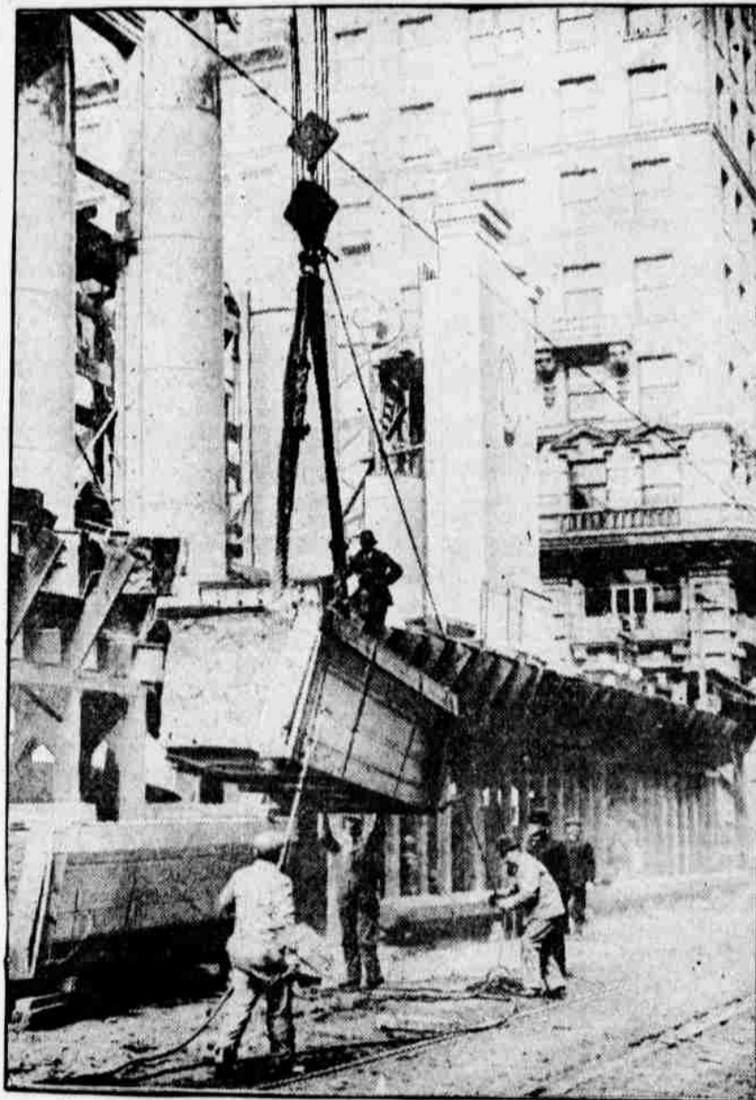
FIFTEEN-TON BLOCK OF STONE BEING RAISED INTO POSITION AT THE NEW HOME OF THE BENEFICIAL SAVING FUND SOCIETY, BEING ERRECTED AT TWELFTH AND CHESTNUT STREETS
