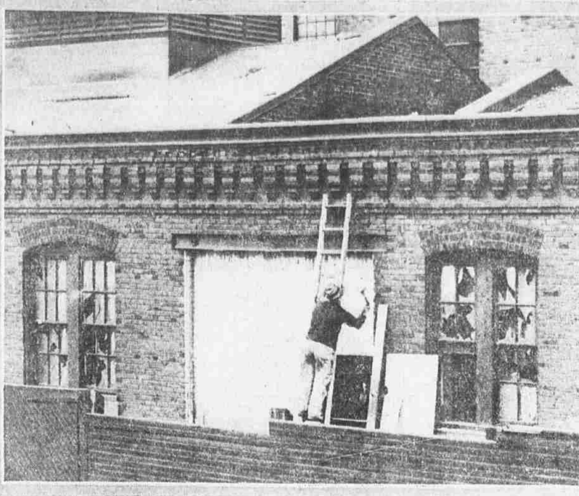
A mysterious explosion this morning in the cellar of Kirschbaum Clothing Company, at Broad and Carpenter streets, damaged the plant and shattered windows in the neighborhood.
