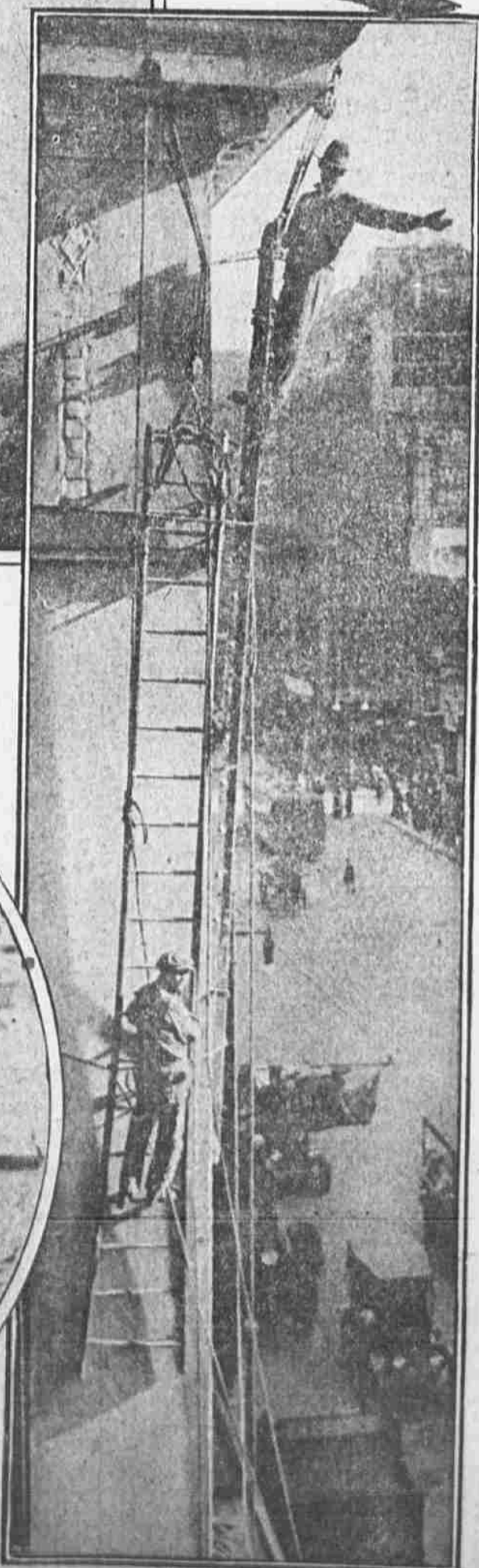
PUTTING UP A SIGN ON THE HIGH BUILDING AT ELEVENTH AND MARKET STREETS IS ONE OF THOSE JOBS YOU PREFER SOME ONE ELSE TO HAVE
