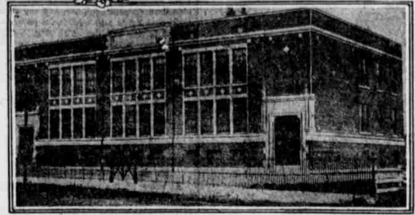
Above is the Kinsey School, at Sixty-fifth avenue and Limekiln pike; below, the Franklin, at Crescentville, which are two of the new buildings erected to reduce the part-time pupils, which last June numbered 24,000
