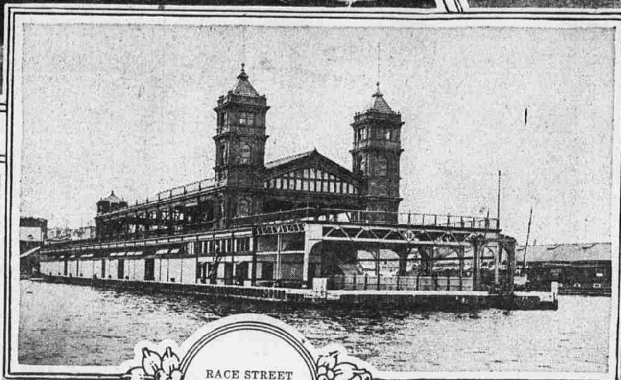
RACE STREET WHARF AND RECREATION PIER
