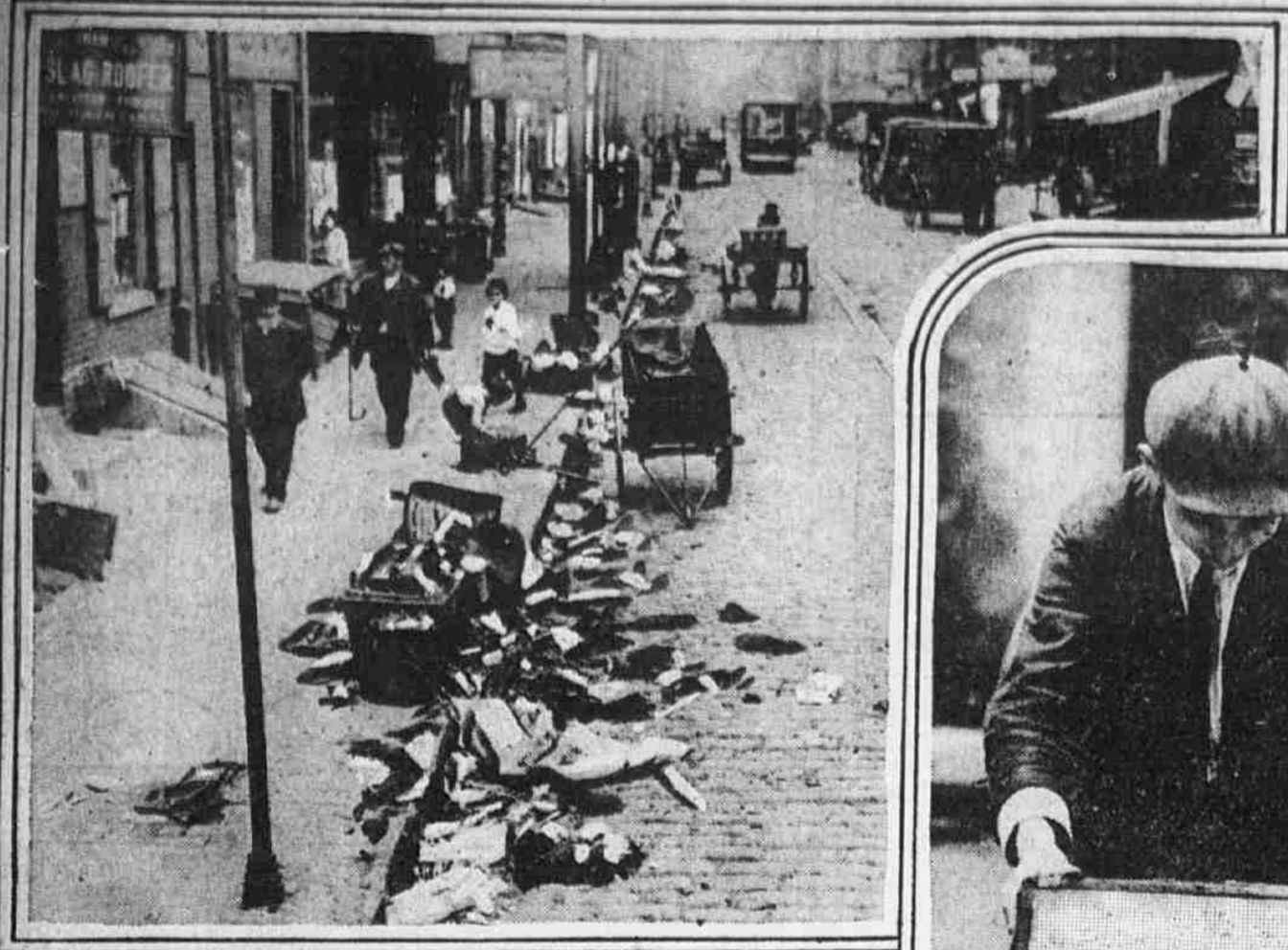
SOUTH 5TH STREET SHOWS URGENT NEED FOR THE CLEANERS-UP
