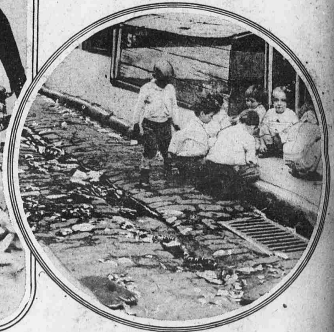
GUTTERS RUNNING WITH FOUL WATER DON'T HELP THE LOOKS OF NORTH 9TH STREET
