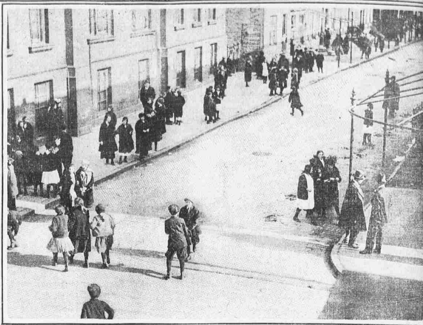
CHILDREN OF PUBLIC SCHOOL FORCED TO TAKE RECESS PERIODS Because a schoolyard has never been provided for the Campbell School, at 8th and Fitzwater streets, its pupils must take to the open streets at recess periods, where they are exposed to all the dangers that street life entails. Repeated efforts of the school heads to have this condition remedied have been in vain.
