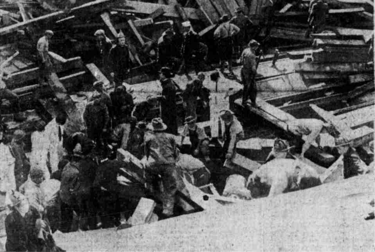
The upper picture shows how a street car was crushed by its 30-foot fall into the hole, killing and injuring several passengers. Below, ambulance workers are shown searching for bodies in the debris.
