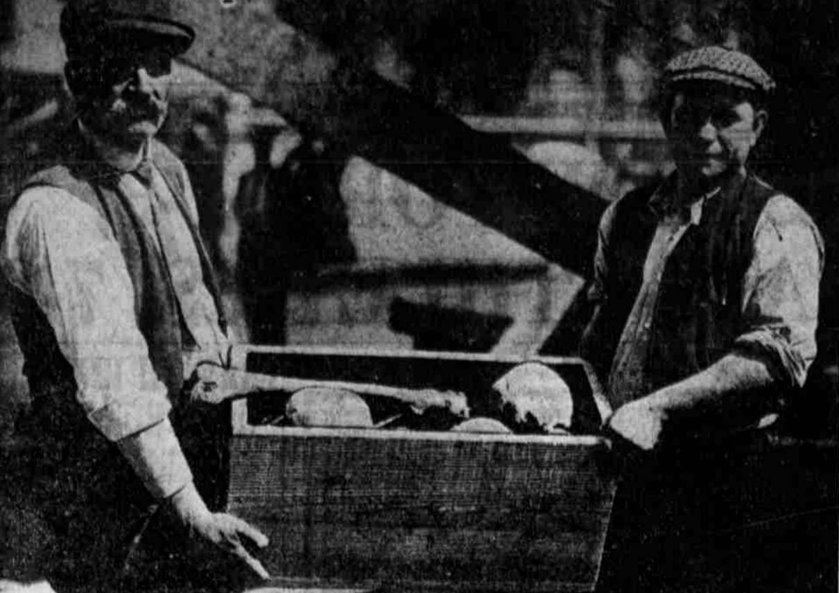
Workmen engaged on the sewer relocation work at the northeast corner of Washington Square, unearthed the remains of seven American war prisoners who died in the British prison formerly at that place.
