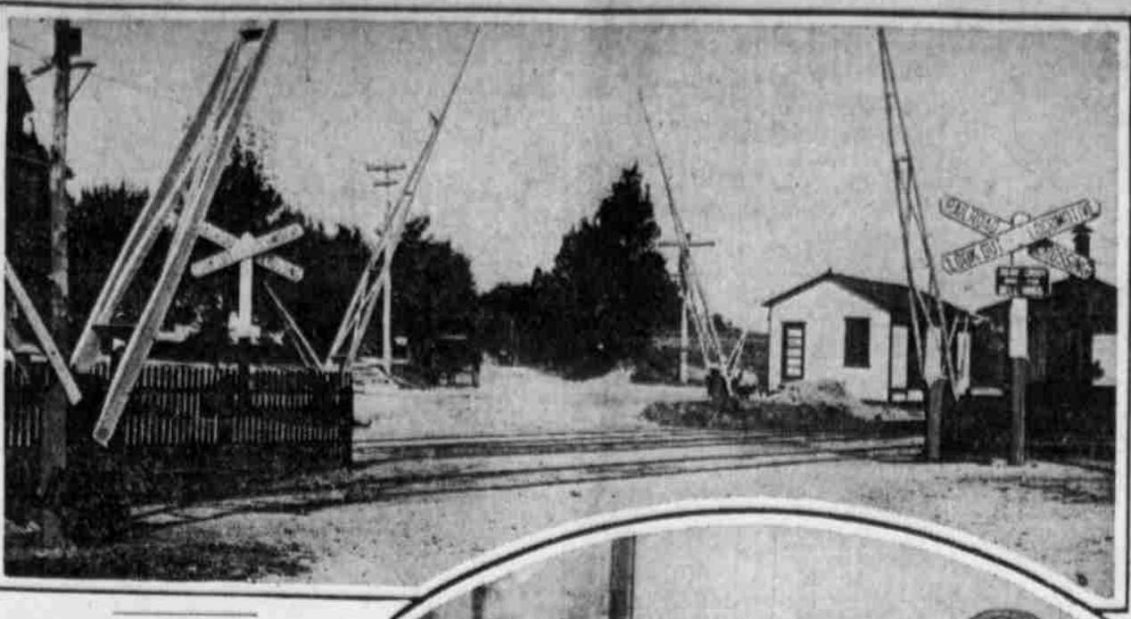
The upper picture shows the Reading tracks at Laurel Springs, N. J., where the express train struck the carriage, virtually demolishing it, as shown below.
