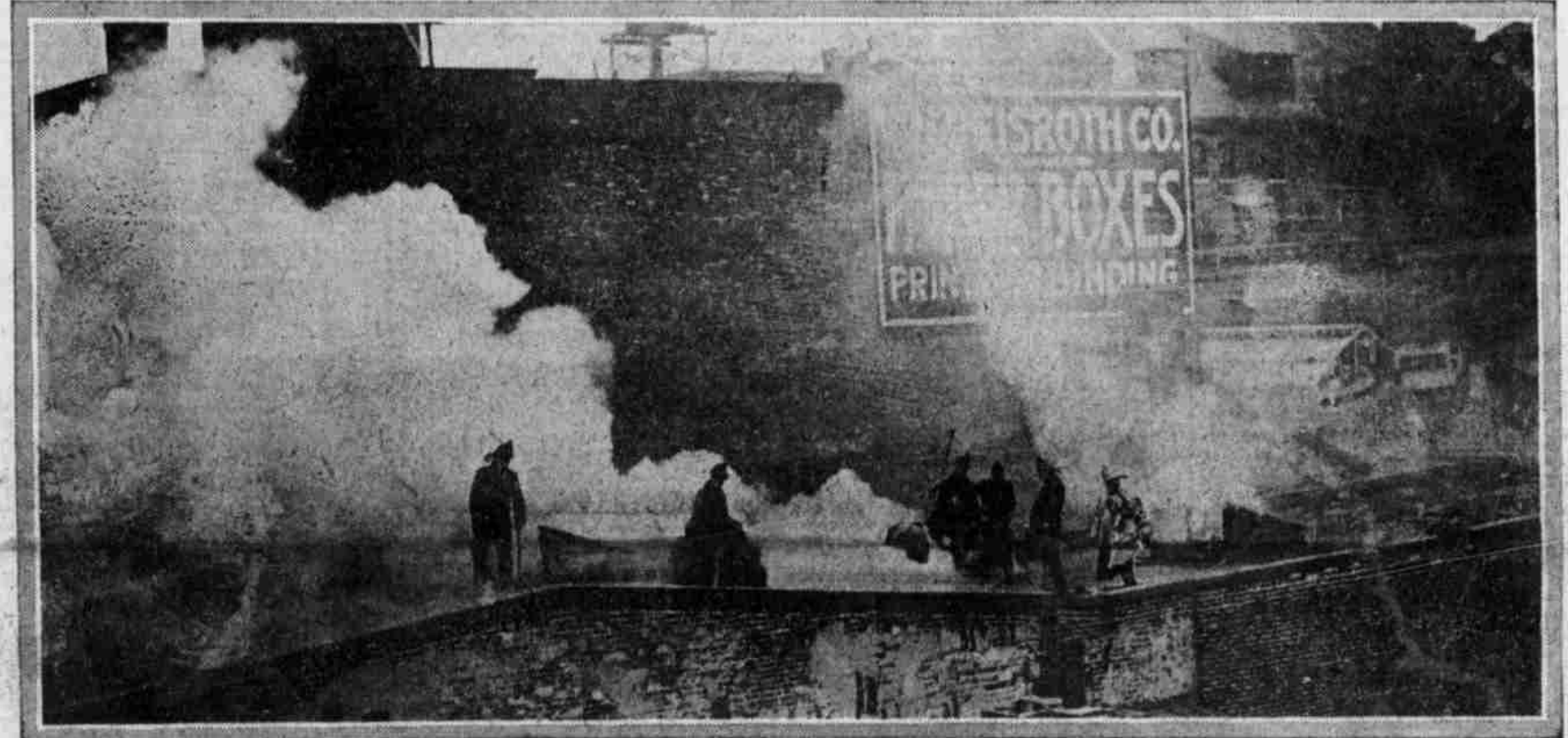
The picture shows the immense volumes of smoke that poured from the paper warehouse at 916 Cherry street today and gave the firefighters much trouble. Two alarms were rung in.
