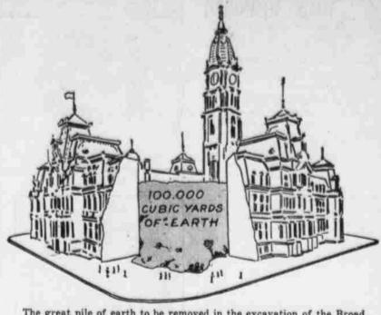
The great pile of earth to be removed in the excavation of the Broad street tube under City Hall would fill the entire City Hall court yard almost to the level of the fifth floor. The City Hall court yard is 200 feet square.
