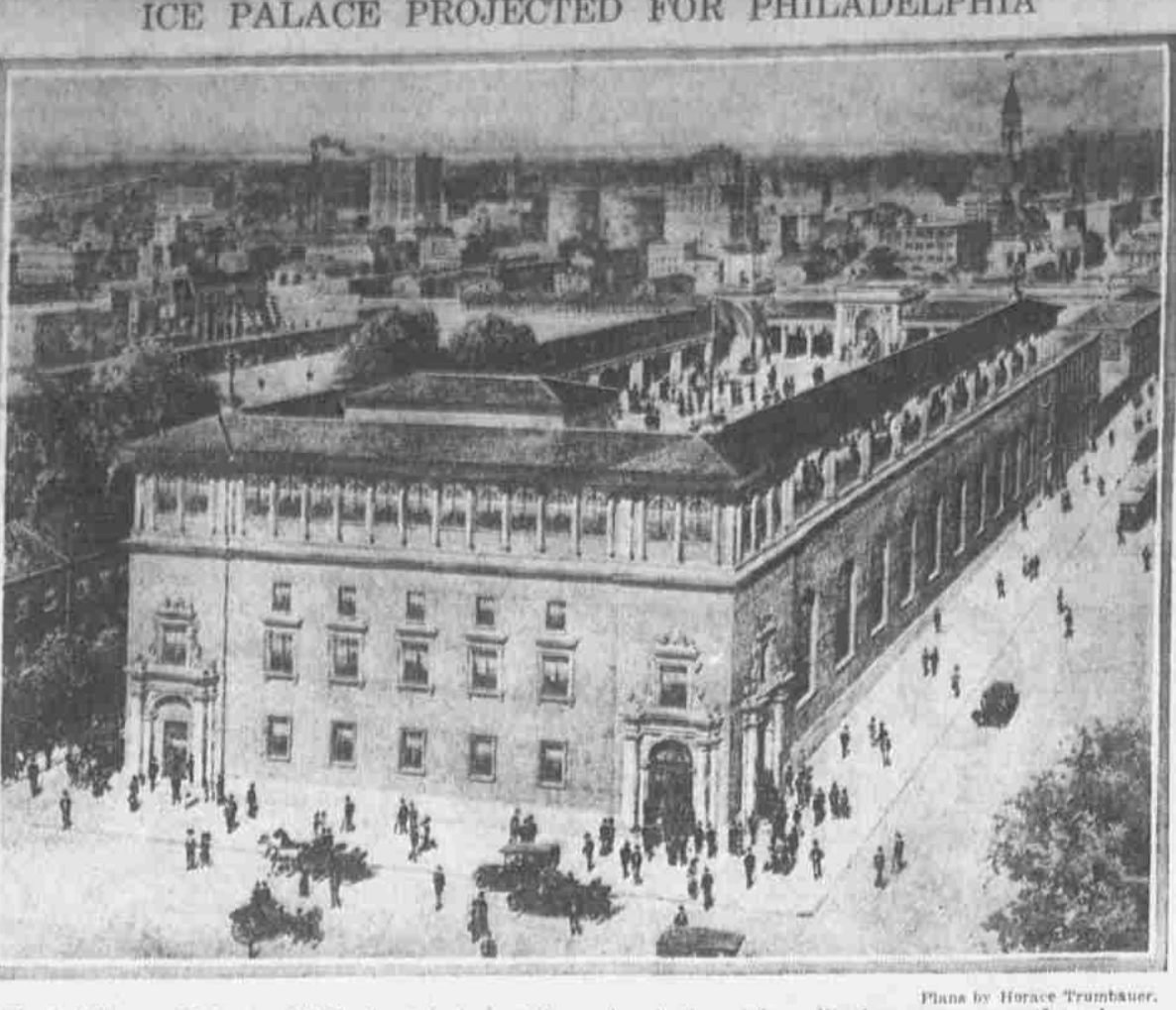
The building at Walnut and 33d street is to contain an ice-skating rink, auditorium, summer roof garden and ice manufacturing plant. It will have a total seating capacity of 6000.
