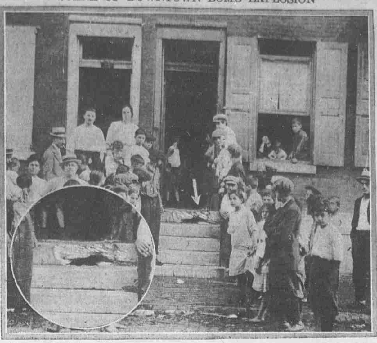
House at 627 Catharine street, where 33 persons were badly shaken up in early morning explosion. The picture shows damage done to front step.
