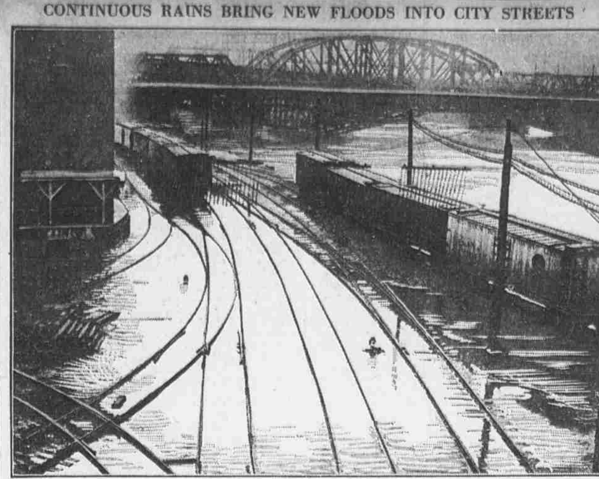
The Schuylkill River overflowed its banks again today, virtually bringing freight traffic to a standstill in the Pennsylvania Railroad yards. This picture was taken at 29th and Chestnut streets.
