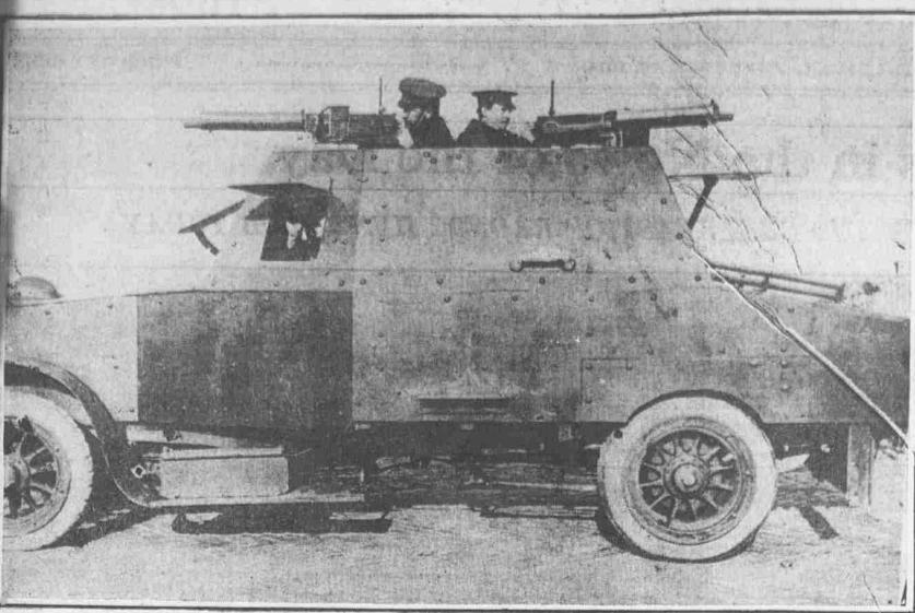
NEW TYPE OF BRITISH ARMORED CAR It holds two Vickers machine guns and is manned by two naval lieutenants.
