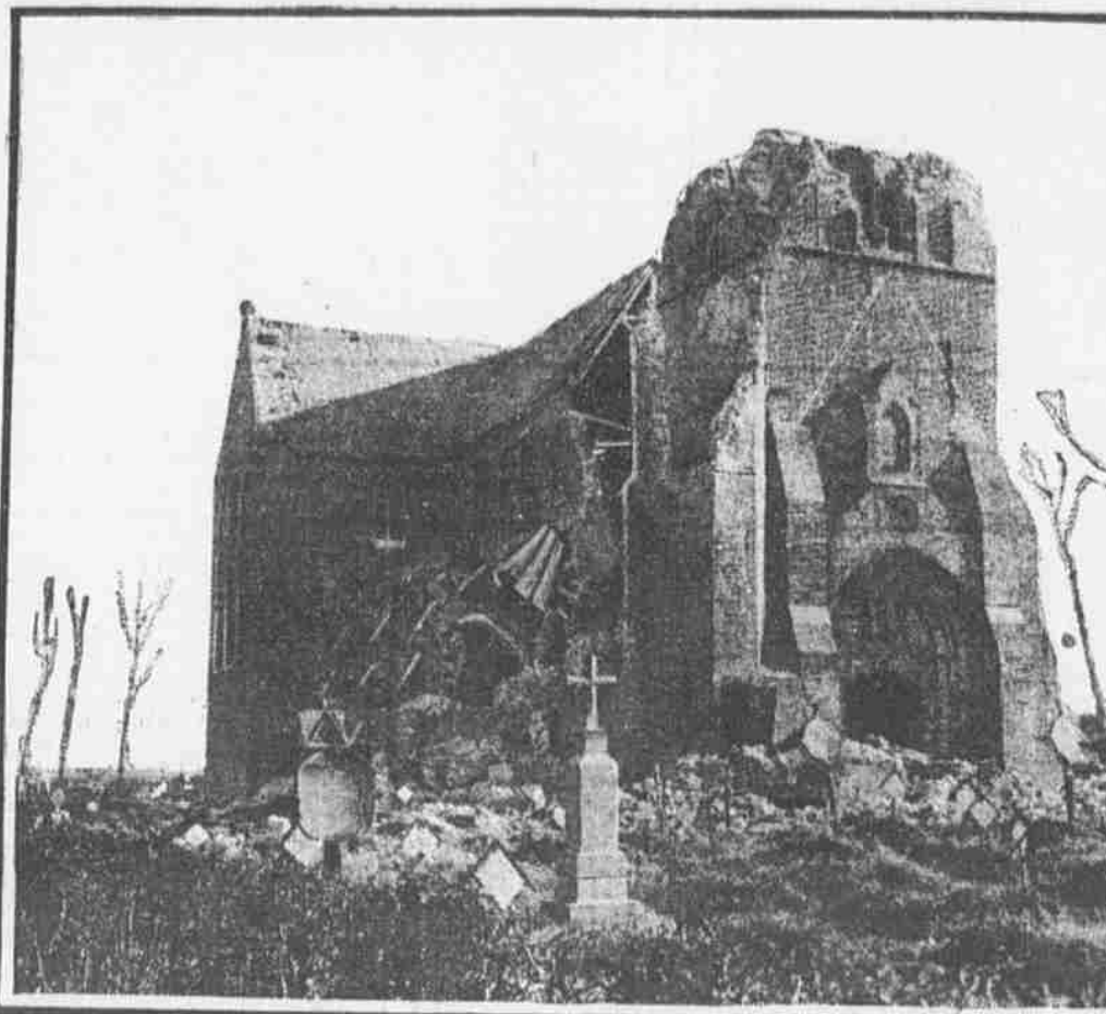
NIEUPORT'S 'MINSTER' AS IT LOOKS TODAY This famous old church, a landmark for centuries, quickly crumbled in the desperate artillery battles that centred around the head of the Yser Canal when the Germans strove to push down the Belgian coast to Dunkirk and other French ports.
