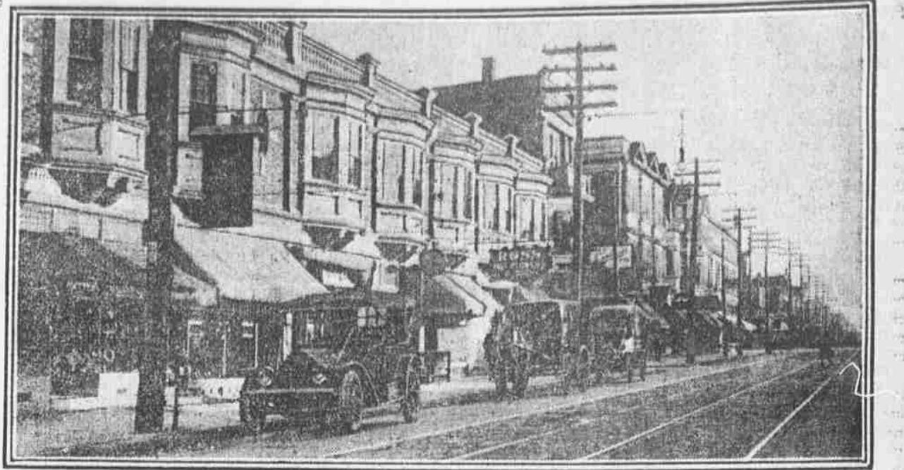
EAST SIDE OF 60TH STREET SOUTH OF MARKET, TODAY
