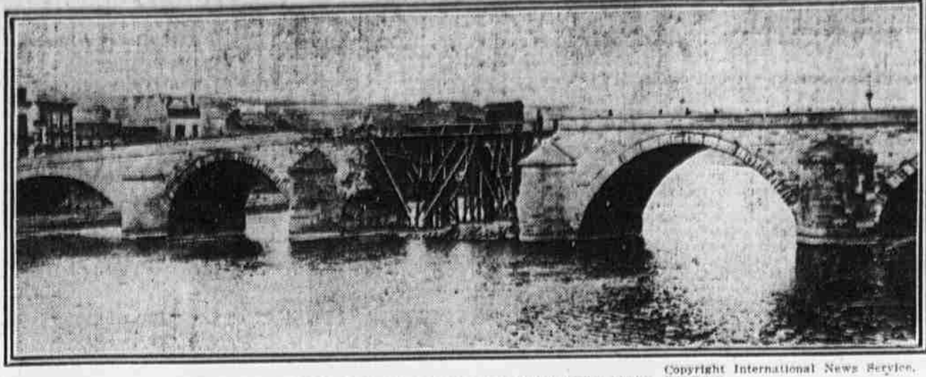
QUICK WORK BY THE GERMAN ENGINEERING CORPS. Bridge at Huy, Belgium, blown up by the Belgians in their retreat and repaired by the advancing Germans.
