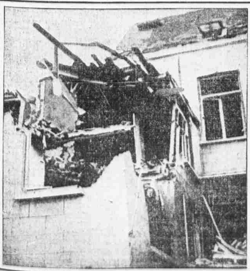
WRECKED BY BOMB WHICH MISSED WIRELESS STATION
