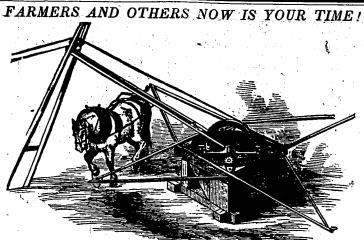
HAINES' IMPROVED LIGHT DRAUGHT HORSE POWER. HE above cut represents the plan of my Horse Power, and the manner in which the Strap passes out over the Horse's back. The Power is very simple in its construction and is arranged to sui
