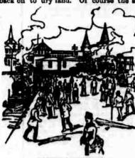
MOVING THE HOTEL. tempt was experimental. To move so large a mass without serious injury, especially considering its great length, it was necessary that the motive power be applied equally at all points of contact with the hotel. The first move was 6 or 7 feet, the second 24 feet, a third 25 feet, a later attempt moved the hotel 614 feet. When the full distance has been traversed, 595 feet of lawn and lanes and flowers will stretch out between the hotel and the
