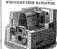
These Heaters are made of heavy Wrought-Iron, w veted together, the only sure prevention against the cape of Gas or Dust. They are easily managed, without any dampers. The Patent Radiator avoids the use and nioyances of drums, and is permanently attached to be Heater. This is the most durable, simple, economi. al, and popular Heating Apparatus ever offered for sale
