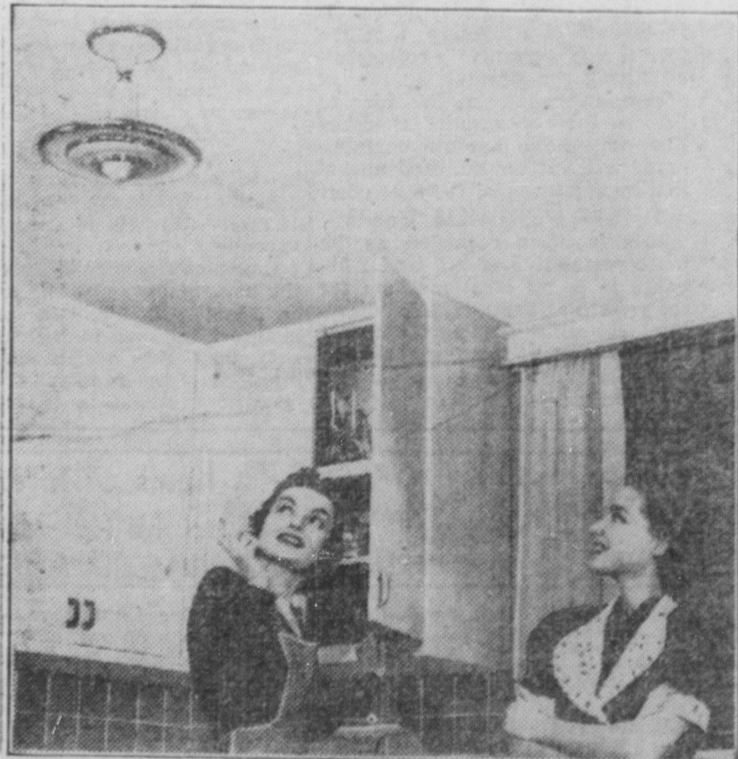
An inexpensive ceiling light for a kitchen or breakfast room is the silvered bowl lamp fixture which can be installed by simply screwing it into an outlet. If you are renting, this type of fixture can be detached and carried along as easily as a portable lamp. Notice in the picture the tubular wall bracket that puts the light right on the work counter.
