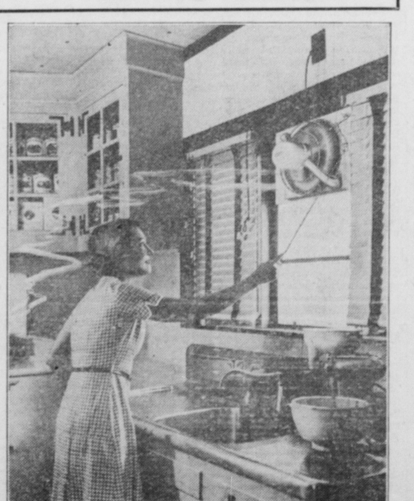
A ventilating fan makes the kitchen a much pleasanter place in warm weather for it keeps the air moving, pushing out the stale air and strong food odors.
