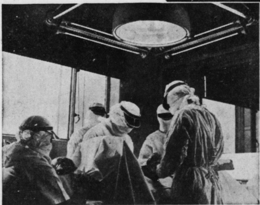
How ultraviolet radiation purifies the air in an operating room, eliminating danger of infection from bacteria in the atmosphere. Note the "sterilamp" in the ceiling, the long tube-like lights.
