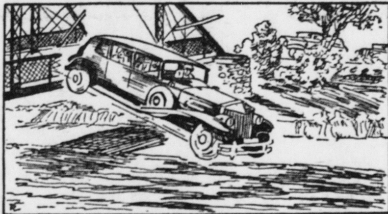
Through the Bridge Railing Into the River.
