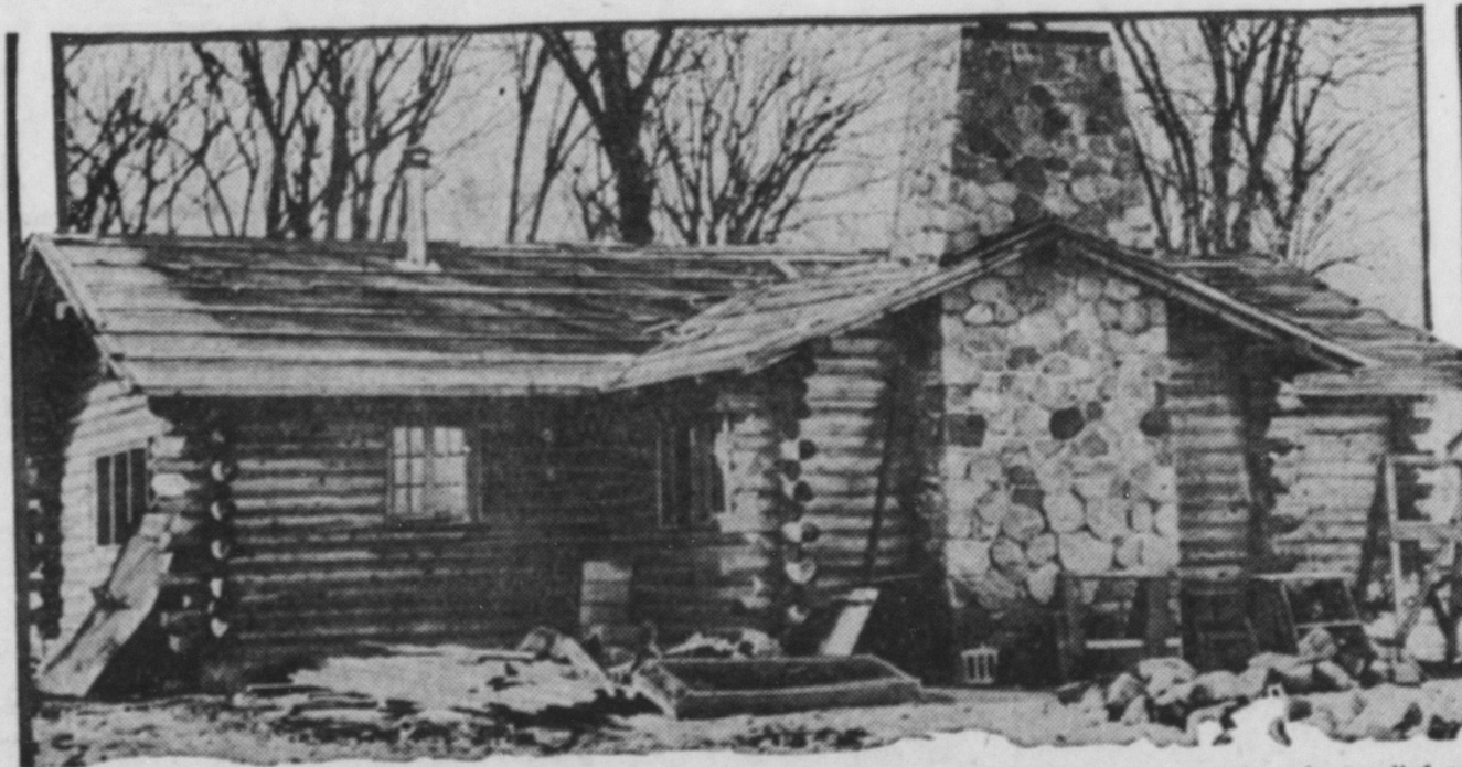
Constructed of old telephone poles, their rotted ends sawed off, this recreation cabin at a transient relief camp near Savage, Minn., cost the state emergency relief $10,900 to build, not including lights, plumbing or interior furnishings, according to testimony presented the Minnesota legislature's investigating committee.
