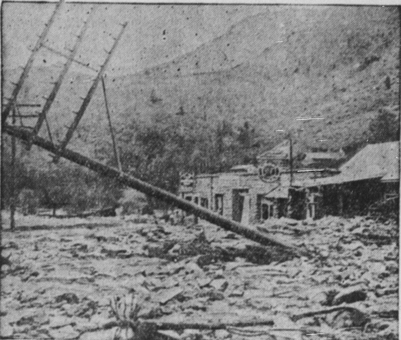
Ruins of the main street of the town of Idlewild, Colo., after a cloudburst swept down Bear Creek canon, taking toll of several lives and doing property damage totaling nearly $1,000,000.
