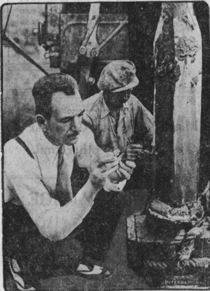
The first well in America in search of helium gas is being sunk in the San Fernando valley near Los Angeles by A. F. Mercet, who is seen above examining matter brought up by the test drill.
