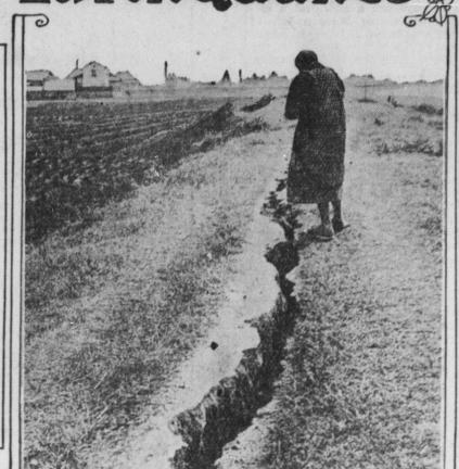
Crack in Filled Ground Caused by Earthquake in Japan.
