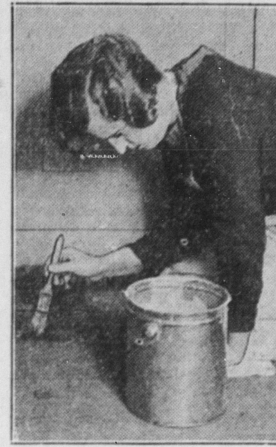
Filling Cracks With Liquid Filler.
