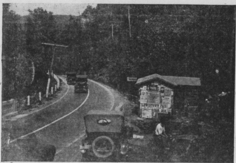
Picture shows concrete road over Centre Hall mountain. At a point one-half mile north of this scene, Richard J. Matthews, of Altoona, was fatally injured, Sunday evening.
