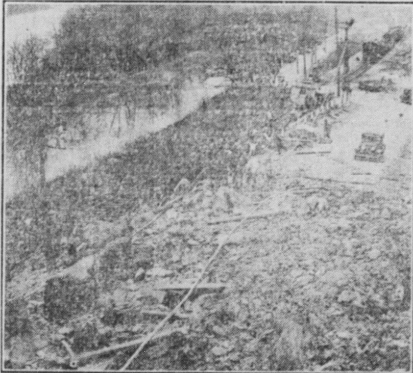
When workmen engaged in a construction project along the Reading-Pottsville Pike set off an unusually heavy charge of dynamite recently, the roadway was buried beneath 150 tons of earth and rock. The Reading-Wilkes-Barre cable of the Bell Telephone Company was torn from the poles and covered by the debris. While emergency crews were rushing repairs, telephone calls were being routed over other lines.
