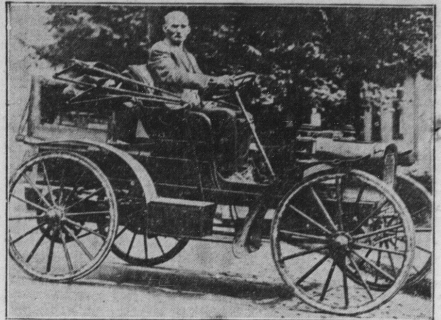
Not many years ago horses ran in terror from this horseless carriage. William F. Wolfe, Upland, Ind., the driver, went more than 250 miles in this speeder to attend the recent Ohio state fair. It was made in 1900, has six speeds forward, and six in reverse, goes 15 miles on one gallon of gas and has a top speed of 10 miles an hour.
