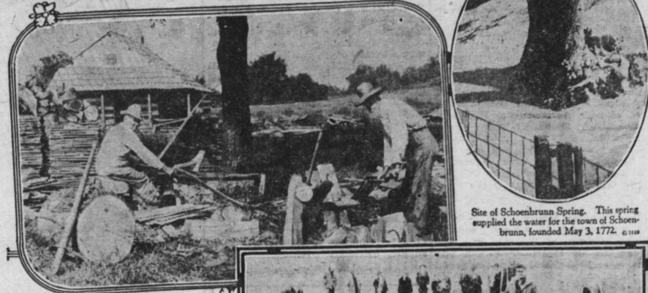
Splitting and shaving shingles—pioneer style—for school house, Sept.-Oct., 1927. Schoenbrunn Memorial Park, near New Philadelphia, Ohio.
