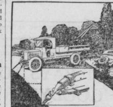
Hooks on Front Springs Permit An. choring the Truck to Lift Heavy
