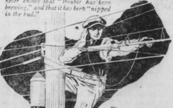
The outside wires, whether they are on poles, or buried under the streets, must be carefully watched. To neglect these tests would spell disaster to the telephone service.
