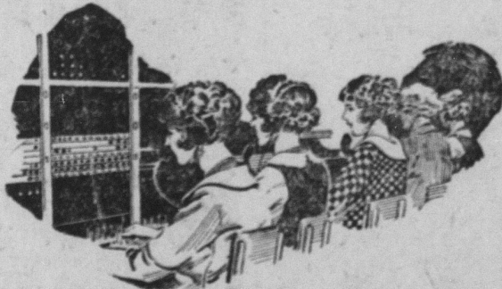
Not for one instant, day or night, holiday or workday, is run the smallest Bell Central Office closed. There are 12,000 Pennsylvania young women who operate the switchboards.
